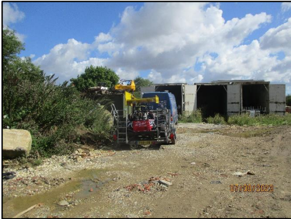
Site yard and containers
