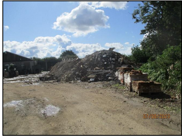
Site yard and steel framed building
